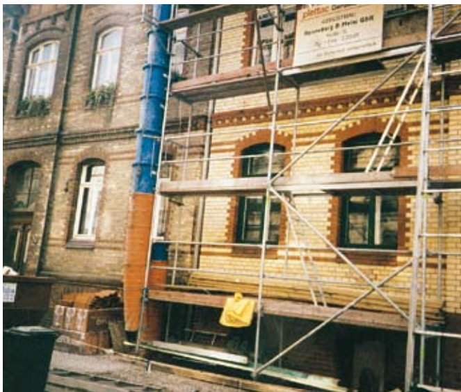
Brick facade, cleaned by waterjetting
