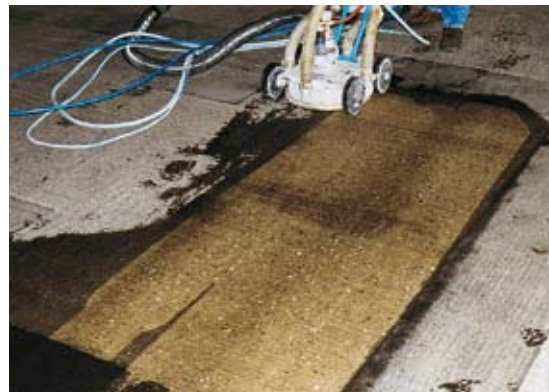
Emission-free cleaning of industrial floors by the Vacu Jet
