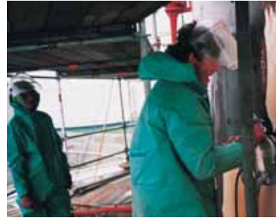
Emission-free surface preparation of superstructures with the Eco Top Rotating Cleaner.
