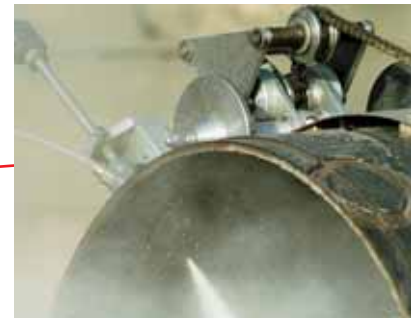
On-site pipe cutting with the 3000-bar abrasive system Eco Top Cutter 3000.
