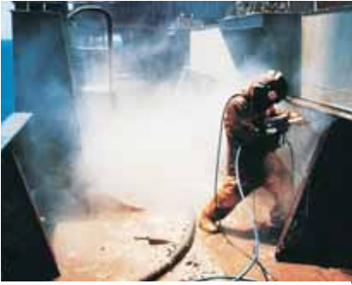
Spot repair on ship hulls with the 3000-bar Modular Gun System.
