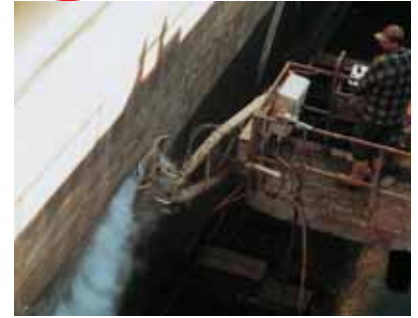
Emission-free mechanised large-scale surface preparation with the mechanical Triple Vacu Jet.
